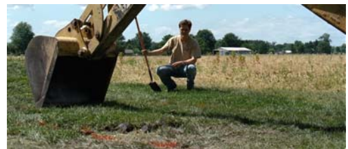
Fig. 1. Curtis, the protagonist of Take Shelter , builds a shelter for his family, risking his job and finances.
